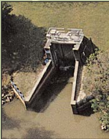
Bayou Darbonne Control Structure
