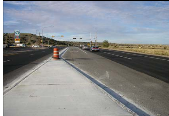
Looking north along NM 30 toward a recently improved intersection adjacent to a convenience store/gas station. The full traffic signal was in place, but not operational, at the time of the audit.
