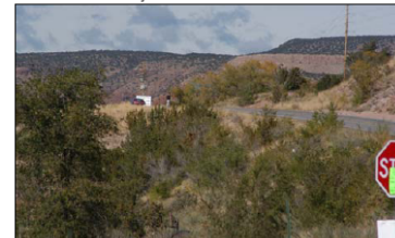
Looking north from Trading Post Road: A roadside embankment is present on the west side of NM4. Drivers leaving the roadway would be unable to recover control of their vehicle on this steep embankment.
