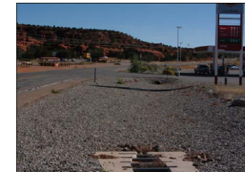
Red Rocks area: The drainage inlet the driveway beyond the gas station sign is a roadside hazard. The near inlet (visible at bottom foreground) has been designed to be crashworthy.
