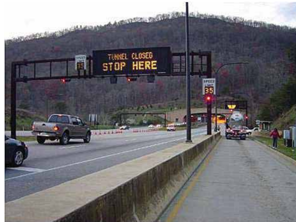
VIEW OF US ROUTE 25E NORTHBOUND APPROACH TO TUNNEL.
