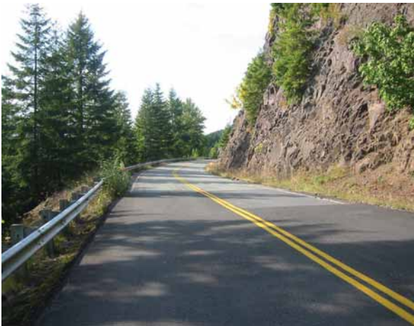
View of the limited recovery area and close proximity of steep rock slopes along Lewis River Road.
