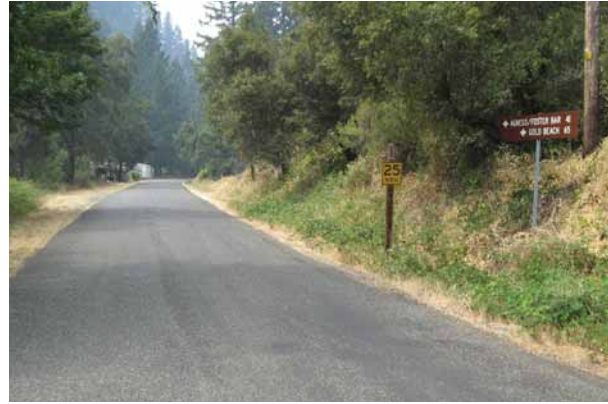
BLM SEGMENT (BLM ROAD 34-8-36), NEAR THE INTERSECTION WITH PEAVINE/SERPENTINE SPRINGS ROAD. A SPEED LIMIT SIGN (25 MPH) IS POSTED AT RIGHT. THE UNMARKED PAVEMENT CAN ACCOMMODATE TWO LANES OF TRAFFIC.
