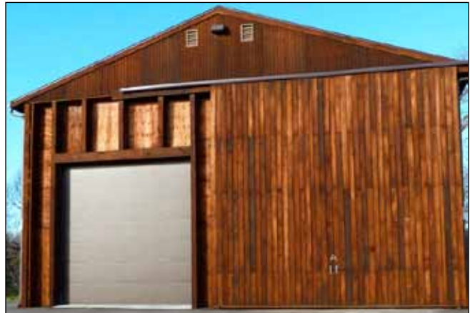
Figure 30. The green color of copper naphthenate tends to weather to brown over time. The photograph on the top is soon after construction and that on the bottom one year later. This wood was pressure-treated.
