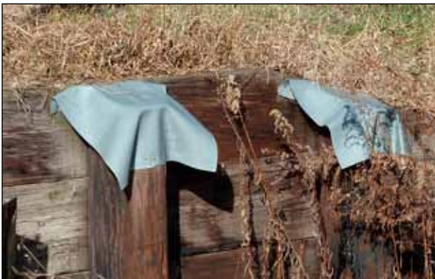
Figure 21. Dense vegetation slows drying after rain and contributes to the deposition of organic matter under and in the bridge.
