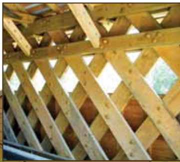
Figure 37. Example in-place treatment of town lattice members below a window opening.
