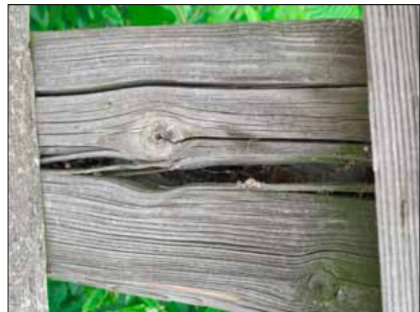
Figure 12. Deep seasoning checks can be an indication of potential problem areas unless the checks formed prior to pressure-treatment.
