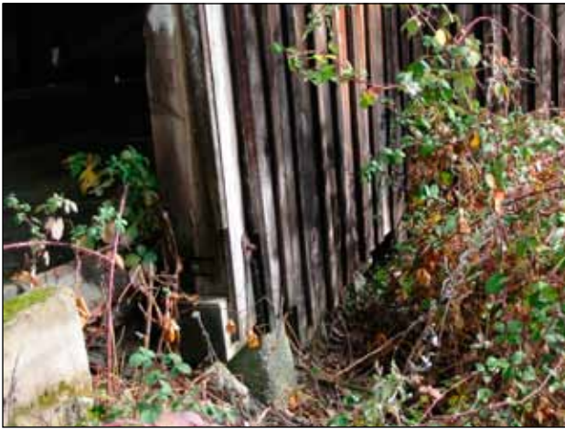
Figure 21. Dense vegetation slows drying after rain and contributes to the deposition of organic matter under and in the bridge.
