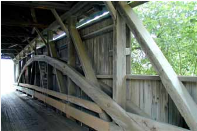
Figure 5. Windows and similar openings in covered bridges provide avenues for moisture entry. Larger and lower windows allow the most access.
