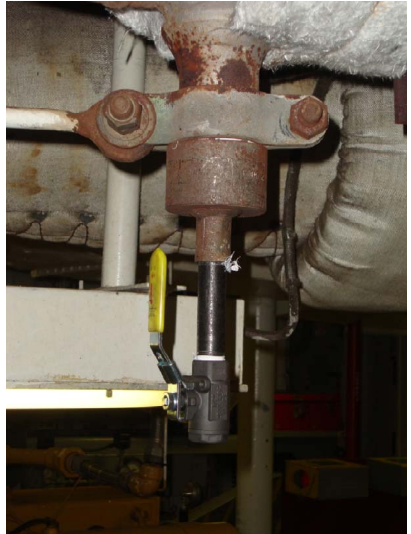
Welded Latrolet and New Drain Valve
