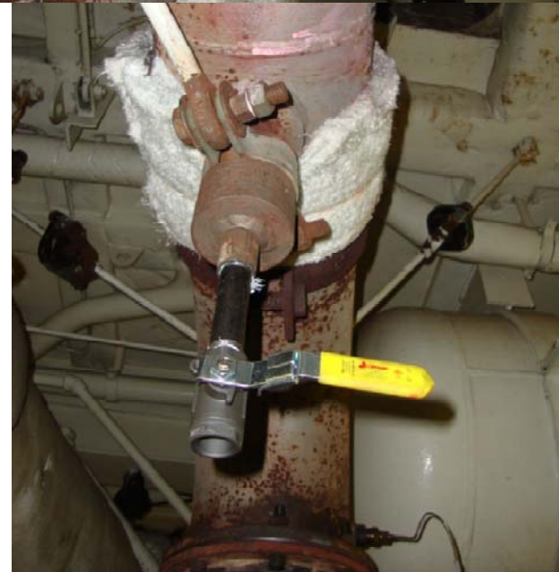
Final Dye Penetrant Inspected Latrolet and Drain Line Renewal
