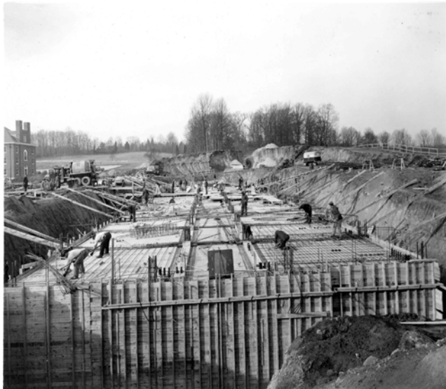
January 1939: Building 6's foundation.
