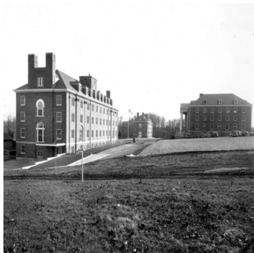
Buildings 1-3 completed Office of NIH History
