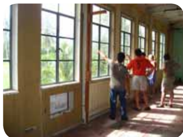
Midway Mall interior: ideal space for offices, classrooms, and visitor services
