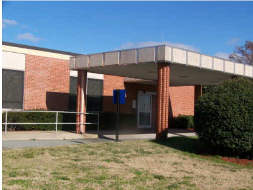
Figure 4.13 Covered Entrance SCI/D Center Long Term Care Center VAMC Hampton, VA
