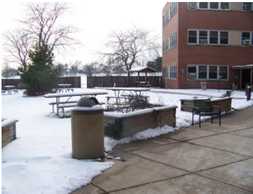
Figure 4.10 Outdoor Walkways and Planted Areas Nursing Home Care Unit VAMC N. Chicago
