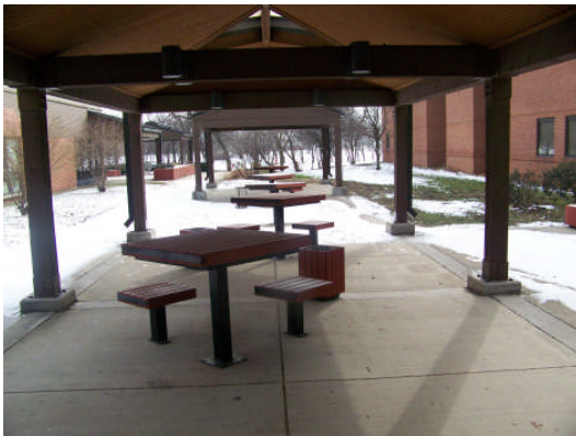
Figure 4.11 Outdoor Dining/Picnic Areas SCI/D Center Long Term Care Center VAMC Hines, Illinois
