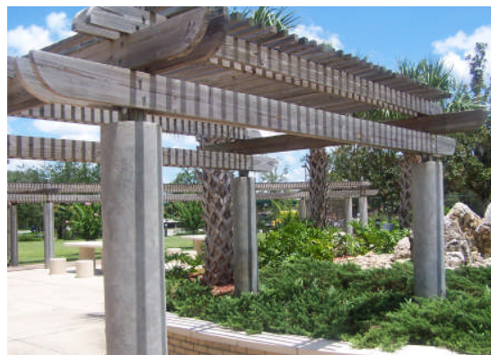
Figure 2.5 Inner Plaza for Social Gatherings SCI/D Center VAMC Tampa, FL
