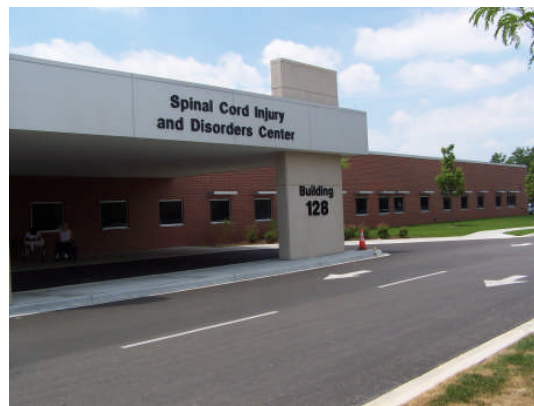
Figure 2.6 Covered Main Entrance and Drop-off SCI/D Center VAMC Hines, IL
