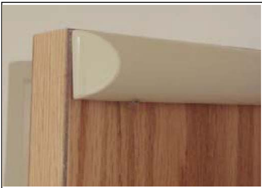
Figure 3.2.6.2: Door Top Pressure Sensitive Alarm
