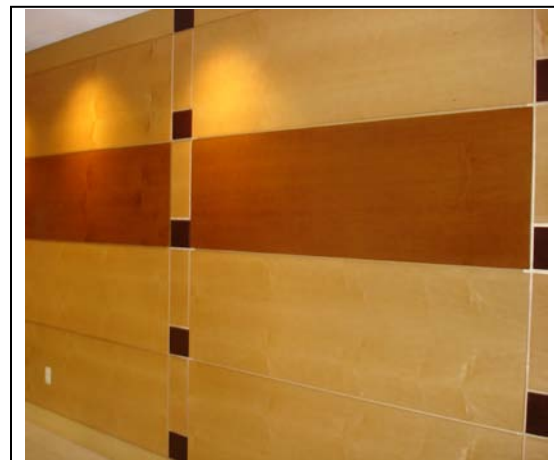
Figure 3.2.7.4: High Impact Panel Wainscot
