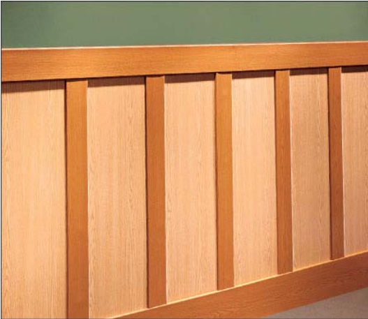
Figure 4.4.4.4: Wainscot Paneling
