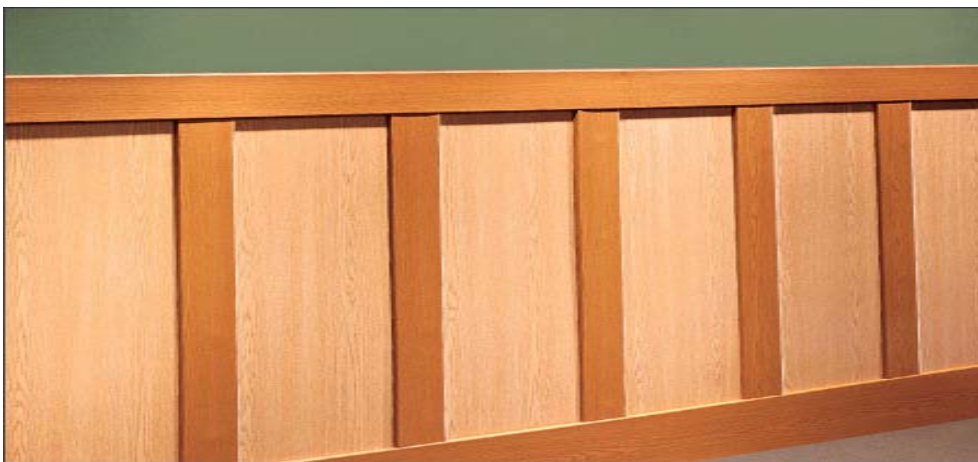
Figure 3.2.5.6: Wainscot Paneling
