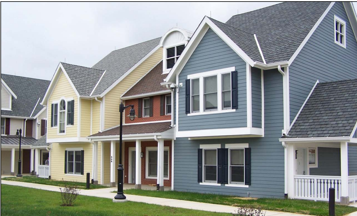
Figure 3.3.1.3 Pittsburgh, PA VA Domiciliary – Detail View of Residential Units Architect: Astorino Photographer: Denmarsh Photography
