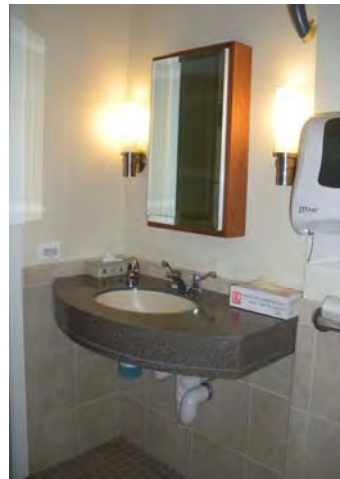
Figure 3-17 Sink in Resident Bathroom The Leonard Florence Center for Living
