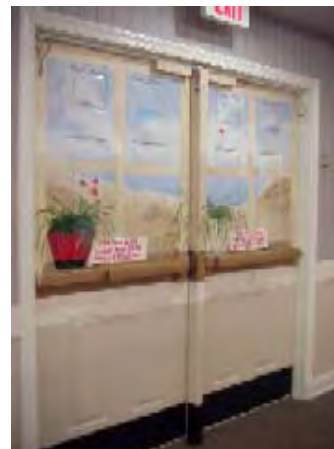
Figure 2-11 Monitored Exit Door with Art Epworth Villa, Oklahoma City, OK
