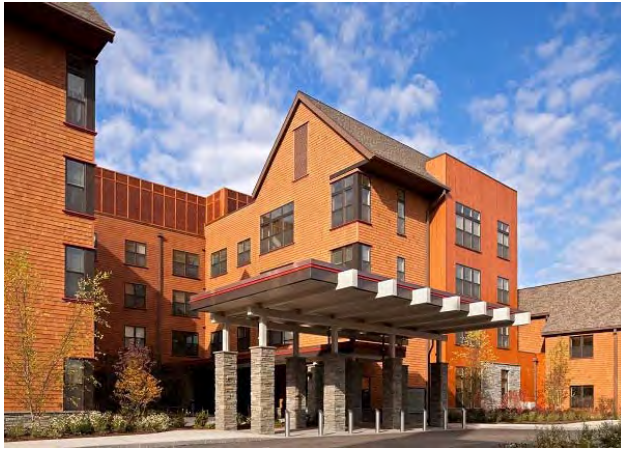
Figure 3-44 Covered Entrance NewBridge on the Charles
