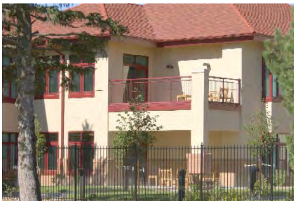
Figure 3-23 Multistory Facility Porch/Verandas CO State Veterans' Home at Fitzsimons
