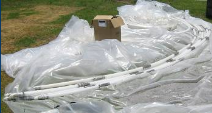
Multilevel Well Construction
