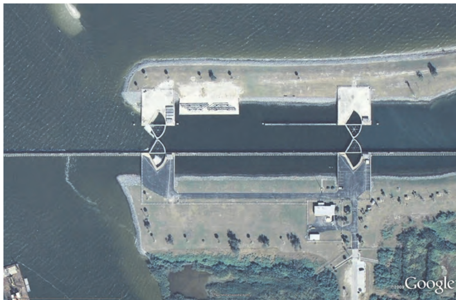
Figure 3. Port Canaveral Lock chamber.
