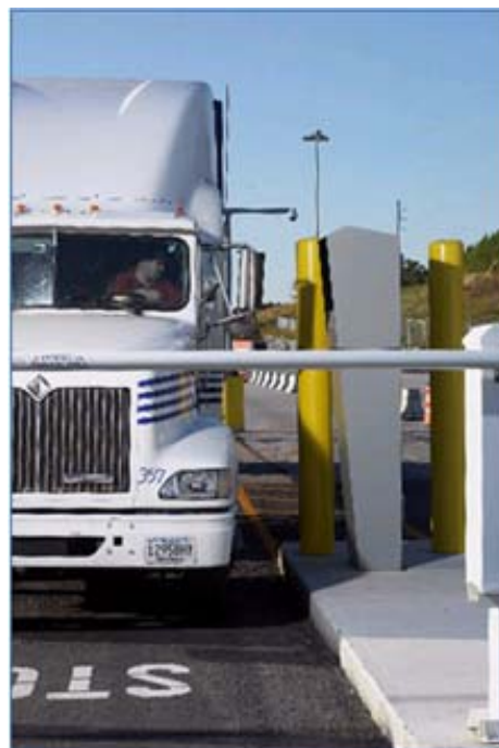
Figure N-14 Automated Gate System
