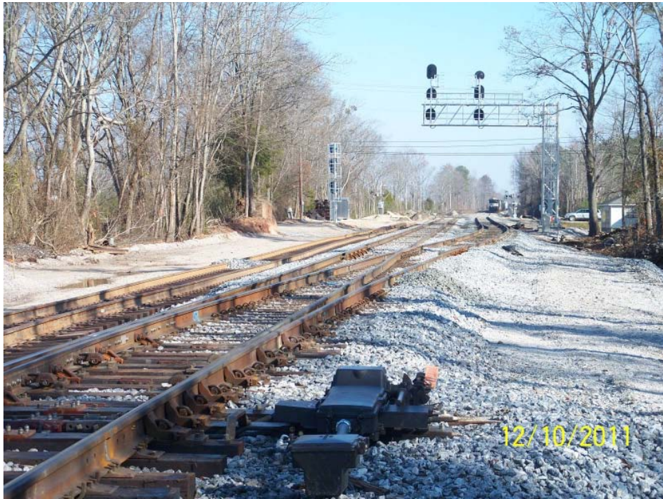
New running track at Kimbrell Cutoff Road Birmingham Intermodal Facility
