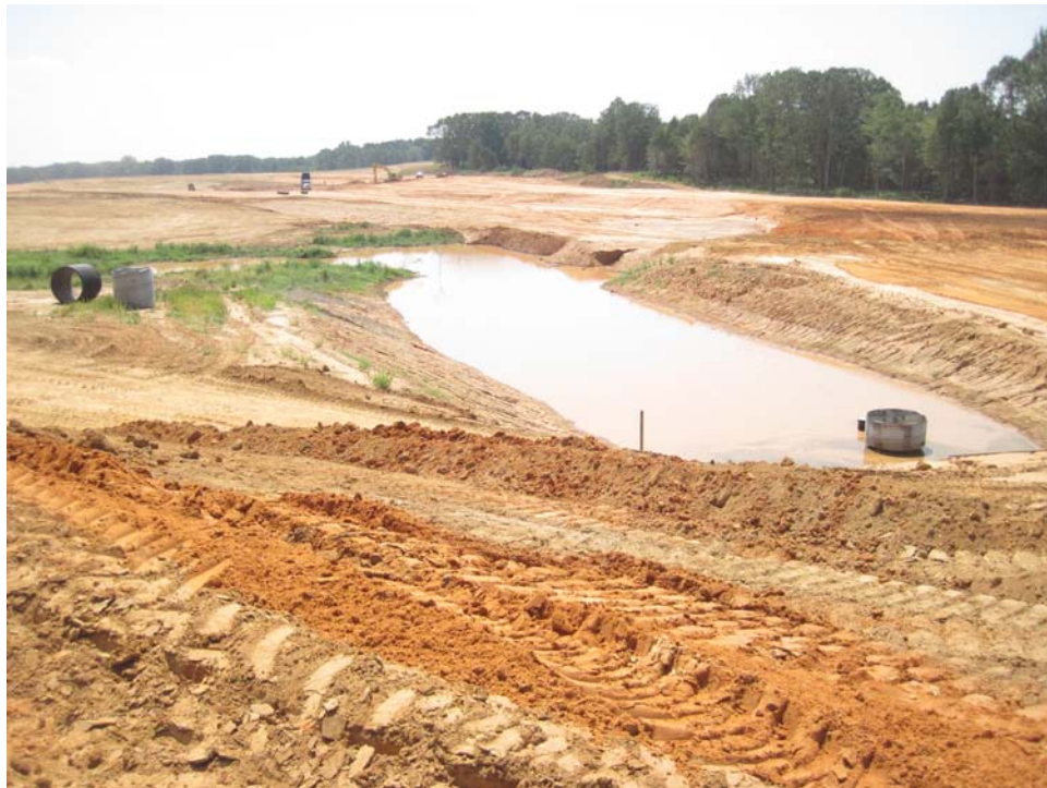
Site Grading (including stormwater management basin) at the Memphis Intermodal Facility
