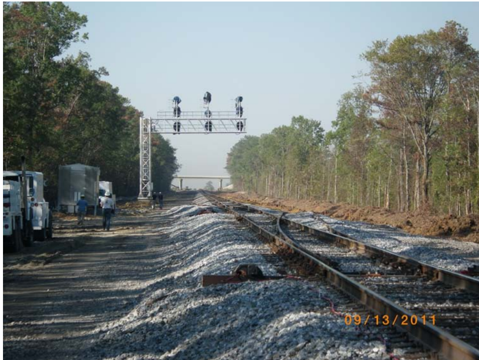
Installation of New Signals at the Birmingham Intermodal Facility
