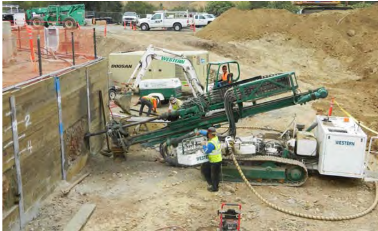
Drilling for Tie Backs
