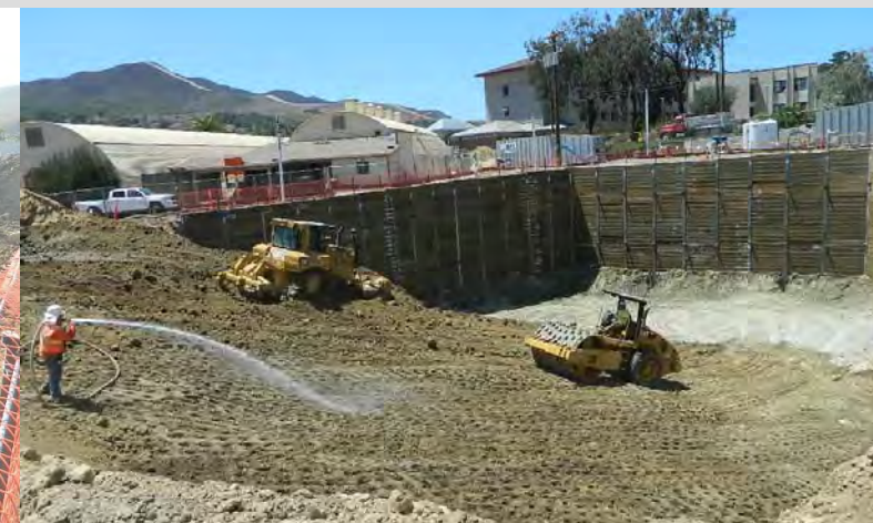
Backfilling
