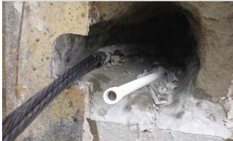
Tie Back Cable and Grout Tube
