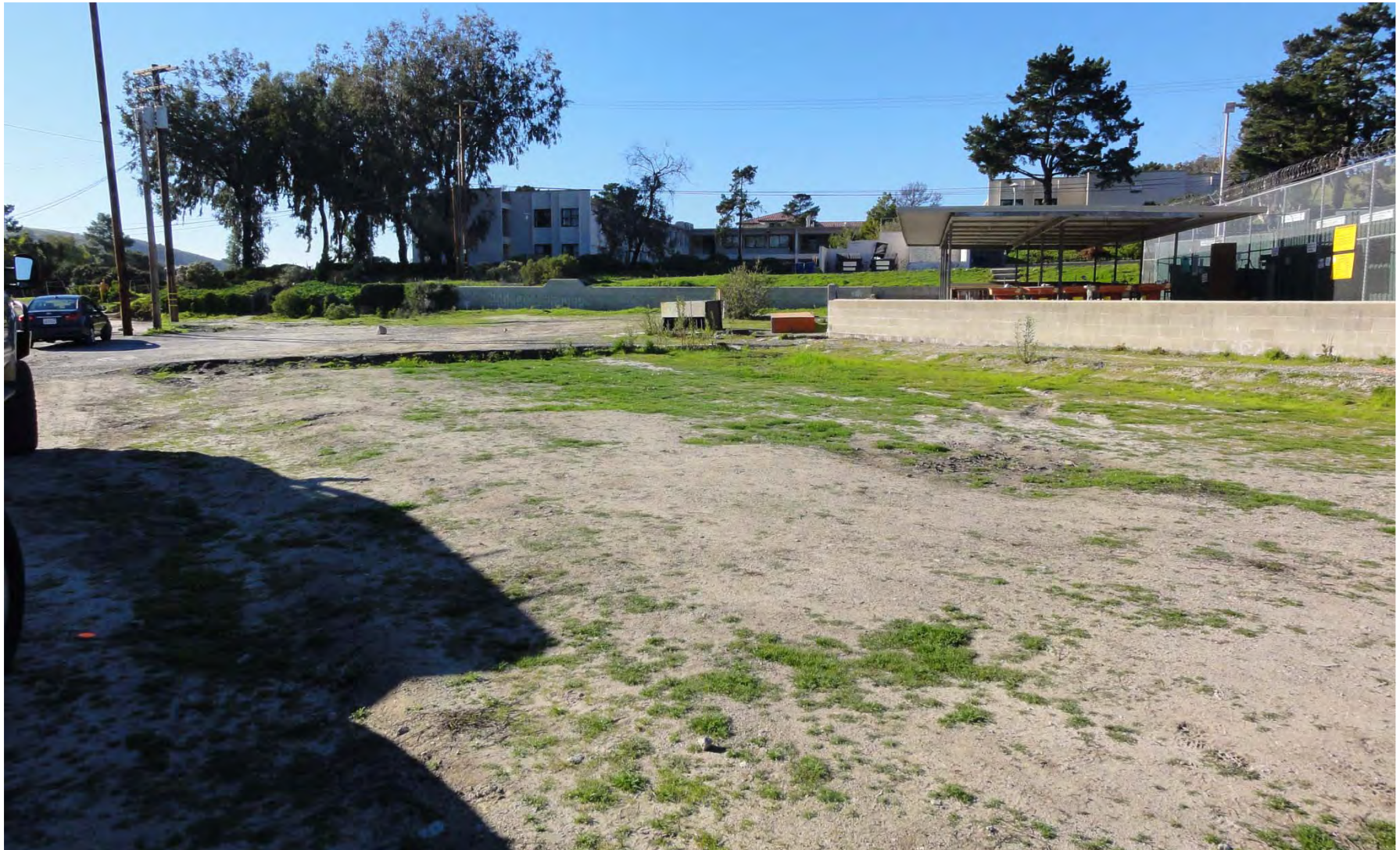
IR Site 33 Pre-Construction
