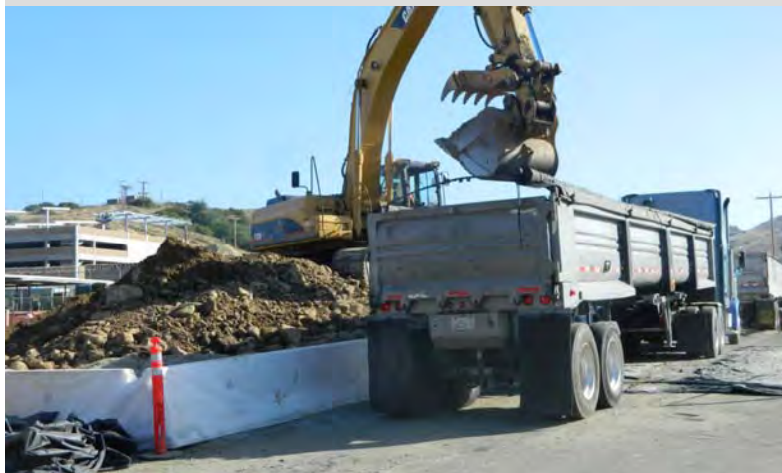
Loading Soil into Trucks
