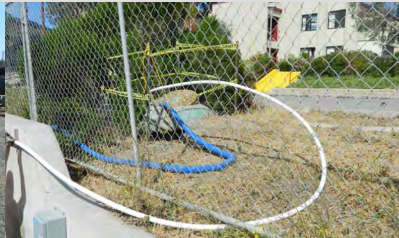
Discharge to Sanitary Sewer
