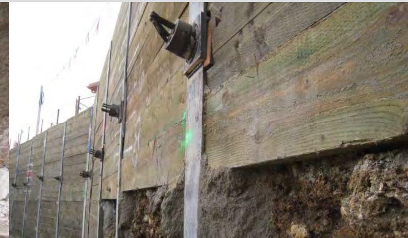
Seven Foot Tie Backs Installed
