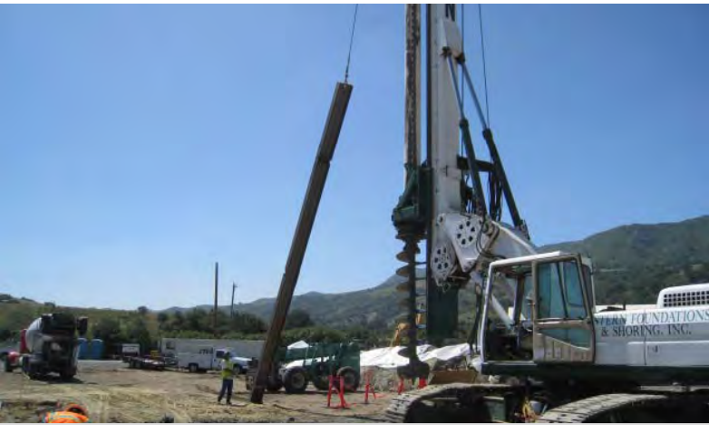
Placing Beam in Drilled Hole
