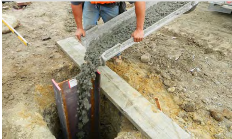
Concrete to Set Piles
