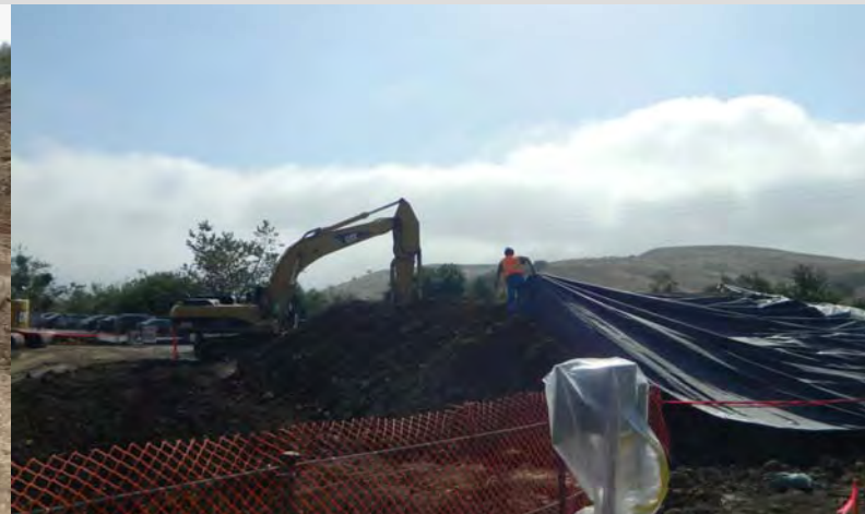
Covering Stockpile at End of Day
