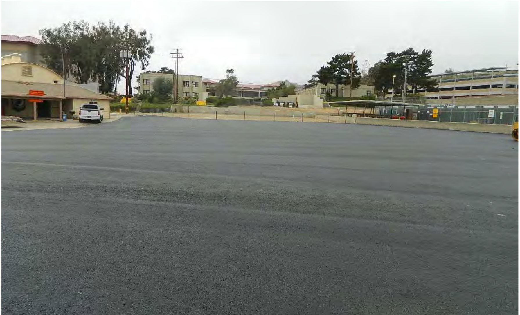
IR Site 33 Post Construction
