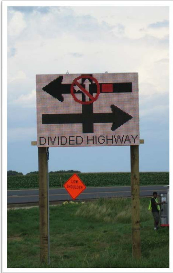
Figure 2. Prototype DIIs as tested at the Minnesota Research intersection at US 52 and CSAH 9 in Goodhue County, MN. The DIIs are 80x112 pixel, 20 mm pitch LED displays measuring 63in by 88in. In the left photo, traffic approaching from the left is more than 7.5 seconds from the crossroads; traffic from the right is less than 7.5 seconds from the crossroads. In the right photo, the nearest vehicle on the left is more than 11.5 seconds from the crossroads; the vehicle approaching from the right is less than 7.5 seconds from the crossroads.
