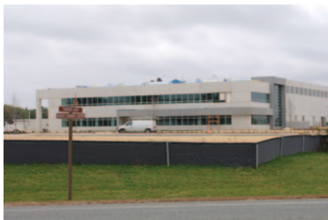
The new VTD facility is located behind the Rodman Laboratory and is expected to be completed by May 2011.
