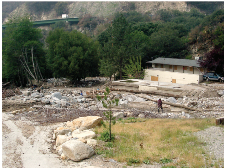
Fig. 1. St. Sophia Church Camp in upper Waterman Canyon near San Bernardino, California. In December 2003, a debris flow triggered from recently burned hillslopes traveled from the bottom to top of this view, leaving deposits and only the foundation of the caretaker's residence. (Photo: Jerry DeGraff, USDA Forest Service)
