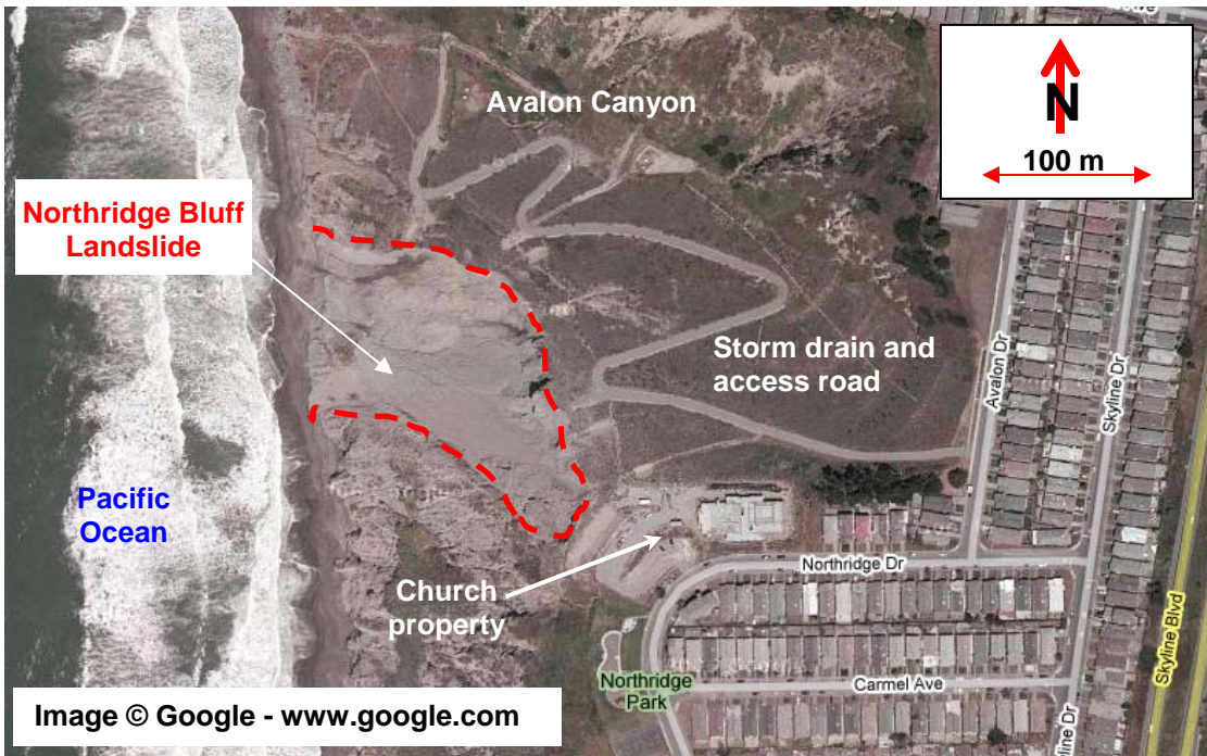
Figure 2. Site map of Northridge Bluff Landslide, Daly City, California showing key features
