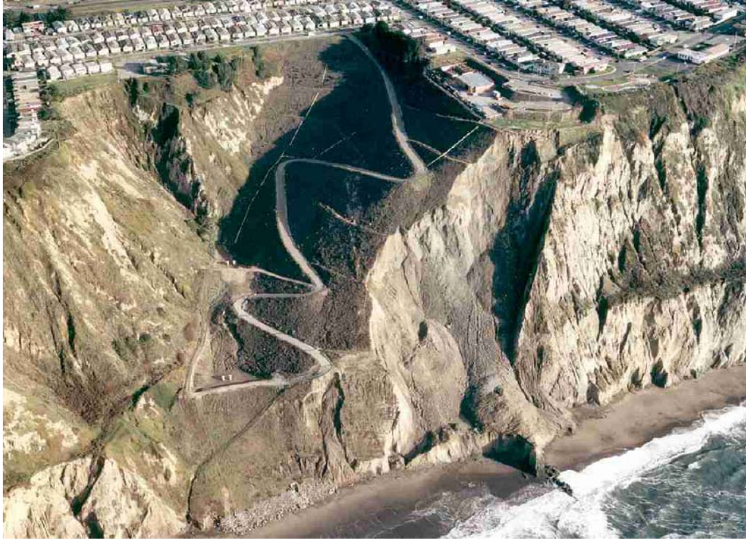
Figure 3. The December 20, 2003 Northridge Bluff Landslide Event (Photo from Cotton, Shires, and Associates, 2004b)
