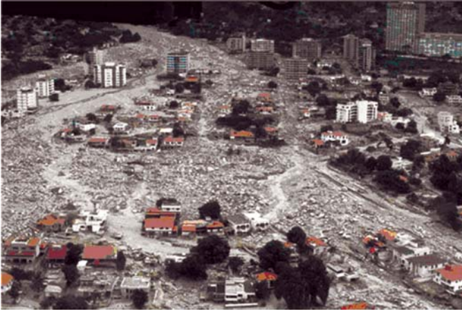
Figure 18. Aerial view of debris-flow deposits up to 5 m in thickness and totaling ~1.8 million m 3 on the fan of the Río San Julián at Caraballeda, Venezuela. Avulsion at the apex caused flow through the center of the fan to the lower right of photograph. (Photograph by Lawson Smith, U.S. Army Corps of Engineers.)
