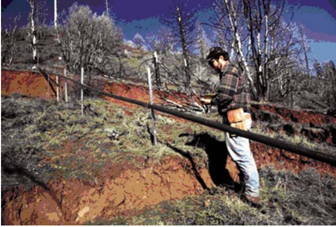
Figure 15. Measuring landslide movement using a surface extensometer. The extensometer crosses several scarps (breaks that expose the reddish soils) at the head of the landslide (Reid and LaHusen, 1998).
