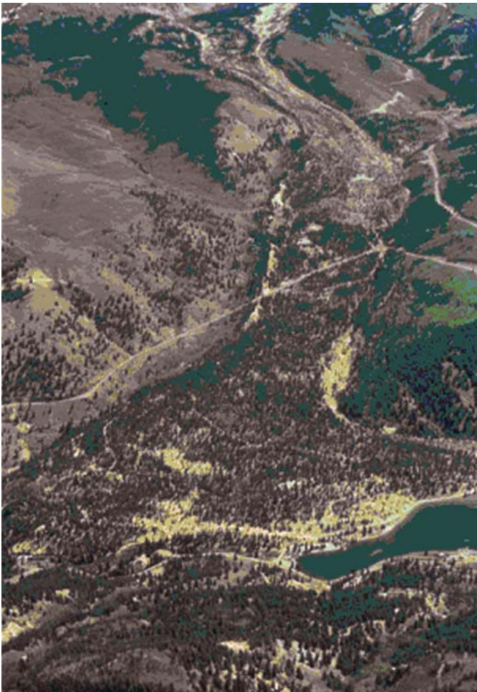
Figure 12. Aerial view of the Slumgullion landslide, Colorado. The inactive landslide extends from the lake uphill to the active toe. Active toe is the prominent light colored bulge uphill from where Colorado State Highway 149 crosses the landslide. The entire Slumgullion landslide is 6.8 km long, covers an area of 4.74 km 2 , and has an estimated volume of \sim 170 \times 10^6 m 3 (Parise et al., 2004).
