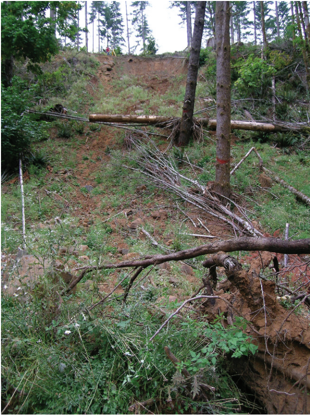
Figure 12. Photo of site 3s5w29-1 taken looking upslope. Plan and profile data of the site are shown in Figure 8. Note boulders from previous retaining wall in the landslide scar, just below yellow total station at top of photo.
