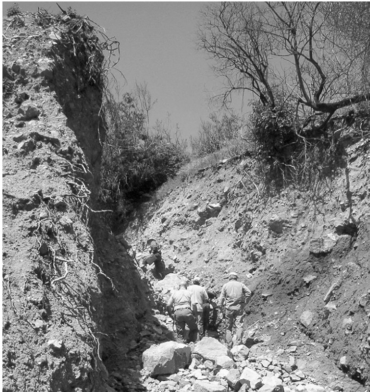
Fig. 7. Deeply incised channel reach with high yield rate. This channel section is in Devore Canyon near San Bernardino, CA, directly above the San Andreas Fault.
