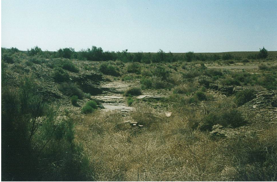
Figure 18.A-13 Spillway channel below No Name Impoundment, location NN-4, looking upstream
