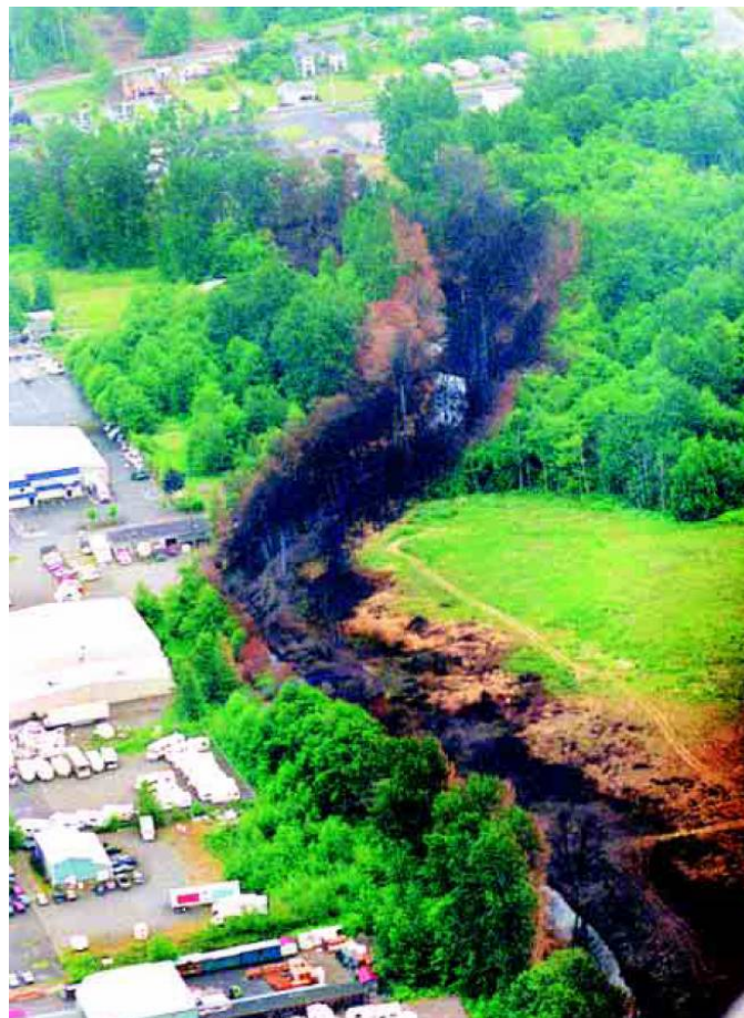
Figure 1.1: Aerial view of resulting fire damage from Bellingham explosion (NTSB, 2002)
