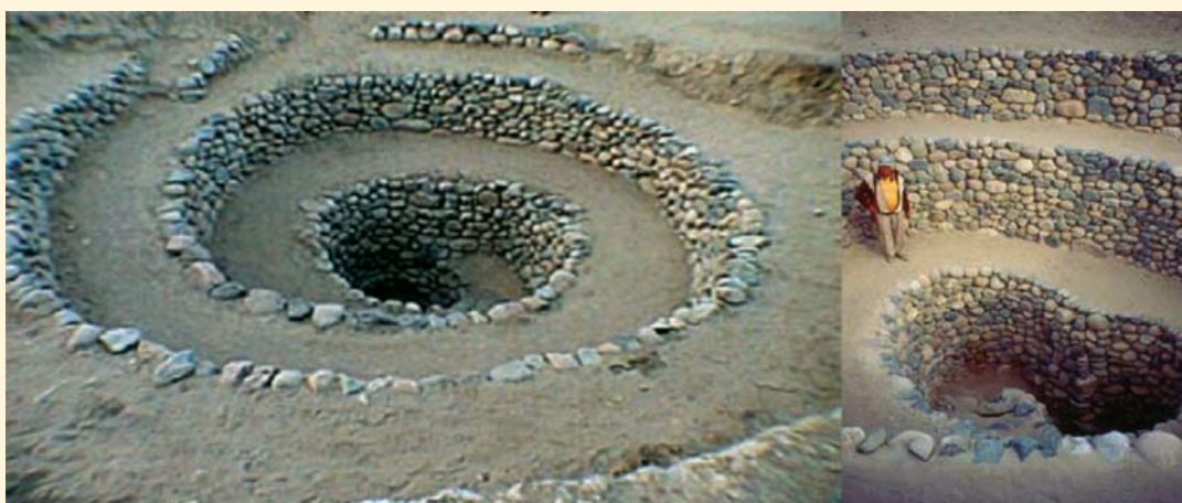
Figure 13.4. Nasca (southern coast of Peru) system of water cropping for underground aqueducts and feeding the phreatic layers.
