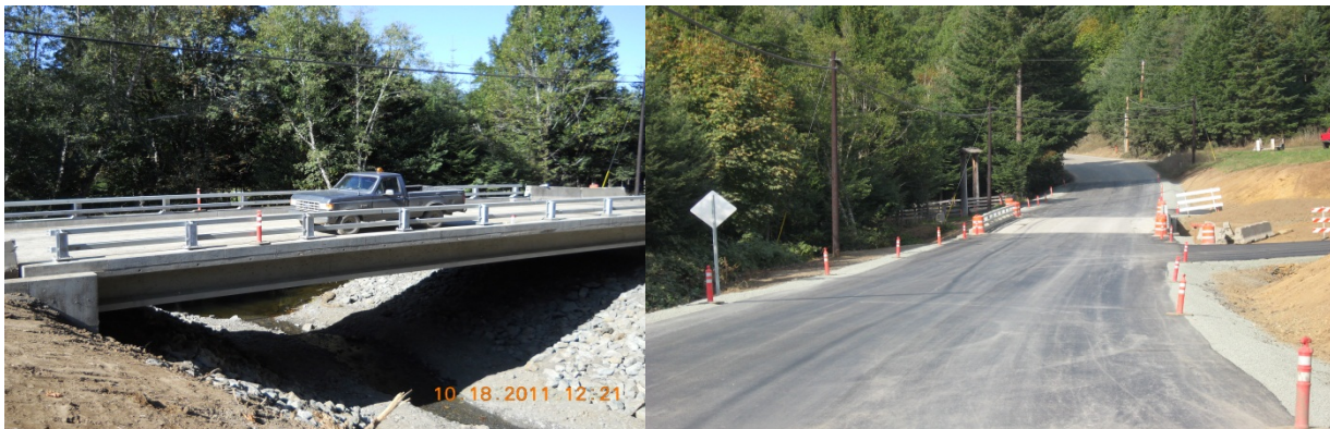
Hayes Creek Bridge and adjacent roadway reconstruction
