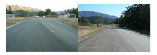
Tidewater has completed placing the first lift of asphalt in realignment area#1, Banner Creek, and half of realignment area#2.
