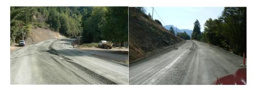
Tidewater has completed placing base rock in realignment area#1, Banner Creek, and realignment area#2. They started subexcavation work and reconstruction of the ditches in the remaining areas of the project.
