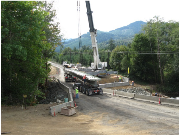
Hayes Creek - unloading girders
