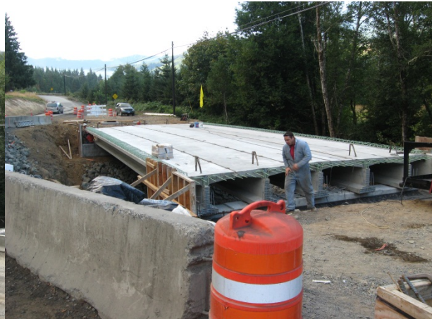
Hayes Creek bridge deck
