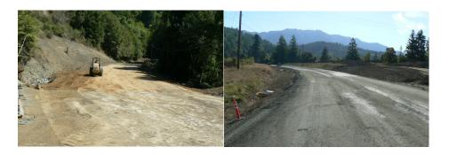
Tidewater has completed placing base rock in realignment area#1 and has finished subgrade at Banner Creek and realignment area#2.
