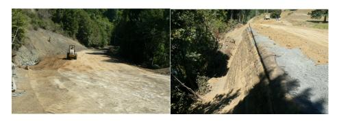
Tidewater has backfilled the Banner Creek culvert and is working on completing subgrade for the road. Tidewater has finished constructing RSS Wall #4.
