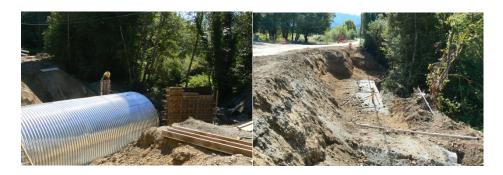
Tidewater poured the headwall finishing the concrete work at Banner Creek this week. Tidewater finished excavating RSS Wall #4 and began preparing the road subgrade in realignment area #1 at the beginning of project. They also paved some of the culvert crossing, getting rid of the bumps.
