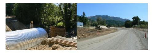
Tidewater installed the culvert at No-Name Creek#2 and poured the wingwalls at Banner Creek this week. Tidewater also backfilled the Mill Creek culvert and removed the one-lane detour.
