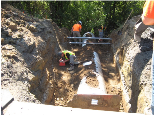
Cross Pipe Installation
