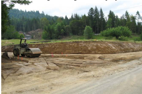
Excavation at Hayes Creek
