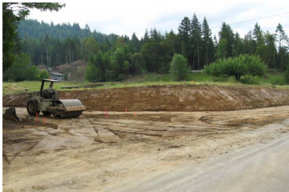
Excavation at Hayes Creek
