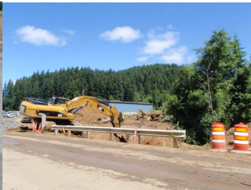
Mill Cr site work
