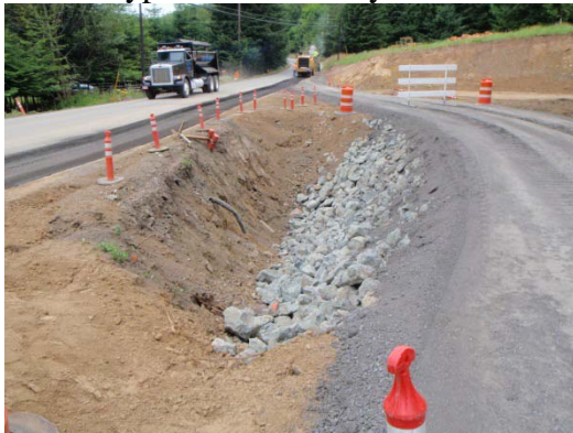
Bypass work at Hayes Cr.
