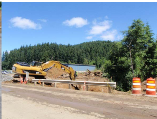
Mill Cr site work
