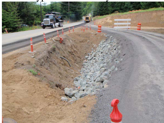
Bypass work at Hayes Cr.
