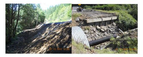
RSS Wall #2 was completed this week. The existing bridge at Mill Creek was also removed and the forms for the downstream headwall where placed.
