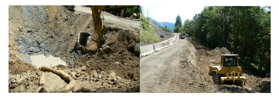
Tidewater Contractors is excavating at Banner Creek preparing to install the new culvert pipe. Excavation for RSS Wall #2 is almost complete.
