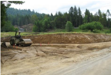
Excavation at Hayes Creek
