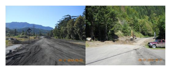
Tidewater Contractors has finished placing the recycled aggregate and is almost ready to start placing base aggregate at the start of the project. Tidewater Contractors installed the diversion pipe at Banner Creek and removed some of the roadway to prepare for removing stage 1 of the existing pipe.
