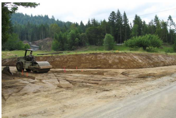
Excavation at Hayes Creek
