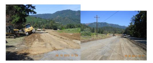
Tidewater Contractors continues preparing the road for paving at the beginning of project. Tidewater Contractors milled the asphalt off of the road in realignment area #2 and placed the material at the beginning of project.
