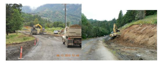
Tidewater Contractors started preparing the road for paving at the beginning of project. They also started finishing the slopes in realignment area #2.
