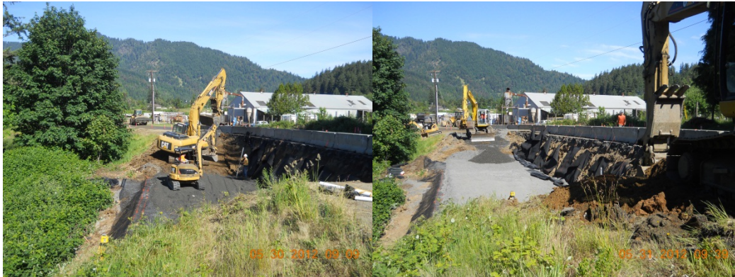
Construction in progress of the Reinforced Soil Slope Wall 1.
