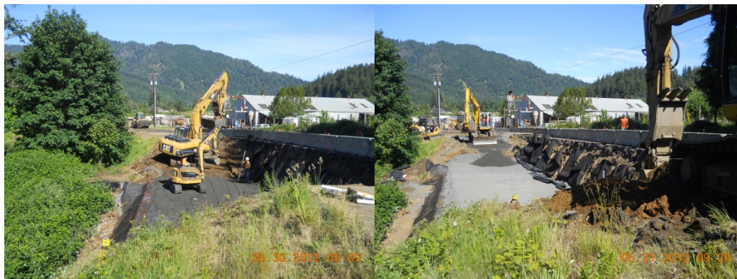
Construction in progress of the Reinforced Soil Slope Wall.
