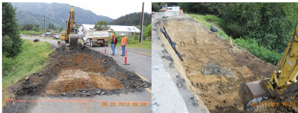
Excavation of the Reinforced Soil Slope Wall.
